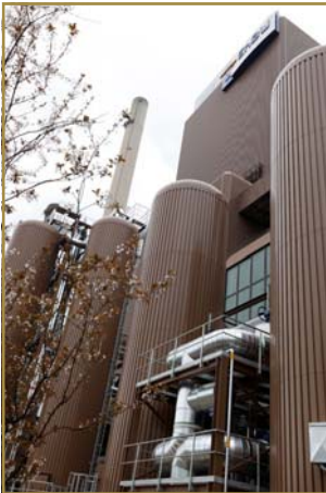
Plant construction for EnBW
