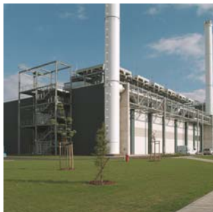
Combined heat and power plants (CHP)
