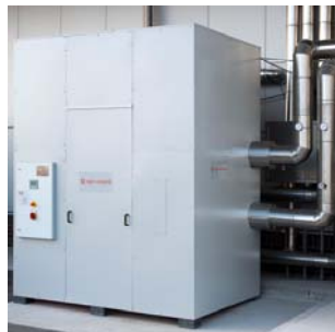
Ammonia-water absorption chiller
