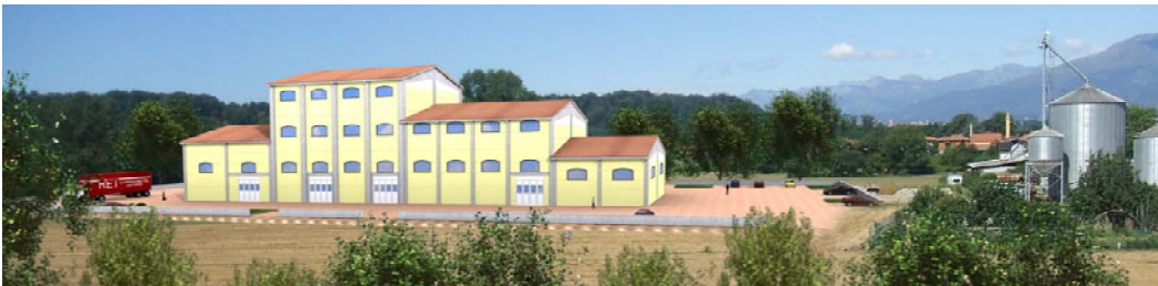
Biomass cogeneration plant of PELLEREI AGO ENERGIA
