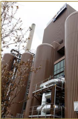
Plant construction for EnBW
