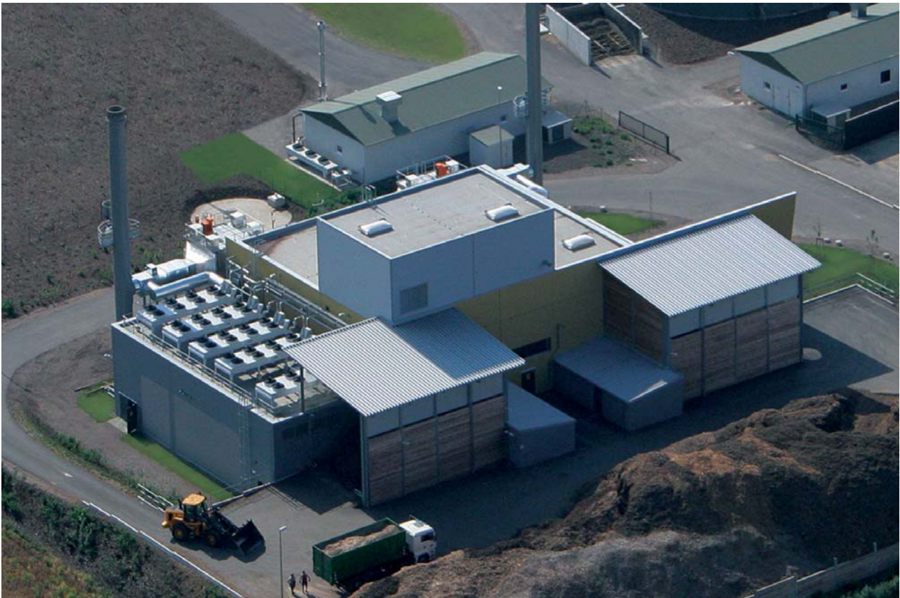
Aerial photo of the Alperstedt biomass cogeneration plant
